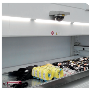
外置式存取口照明灯 External bay lighting
